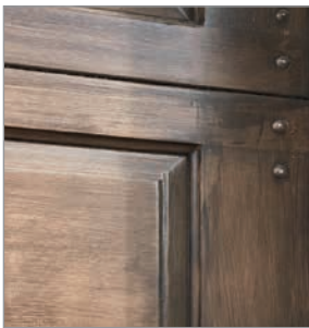
Ends are thru-drilled for carriage bolts
